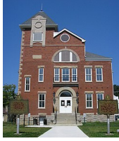
Rowan County courthouse in Morehead
